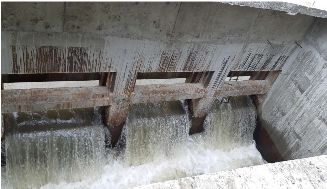
Fig : water entering through orifice.
