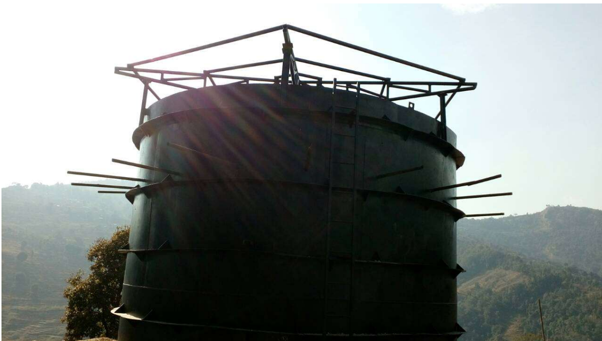
Fig : completed view of Surge
