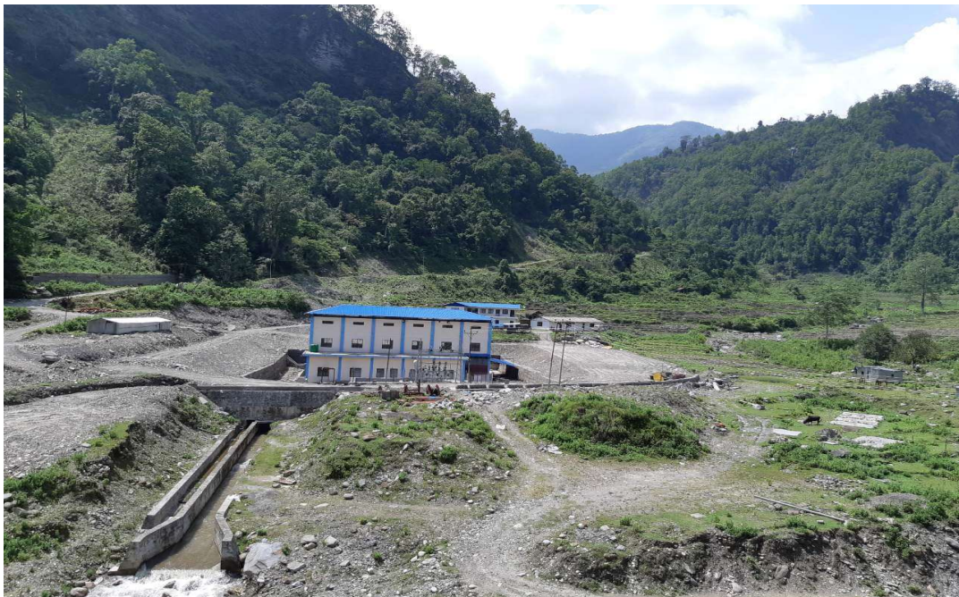
Fig:- Rudi A powerhouse area
