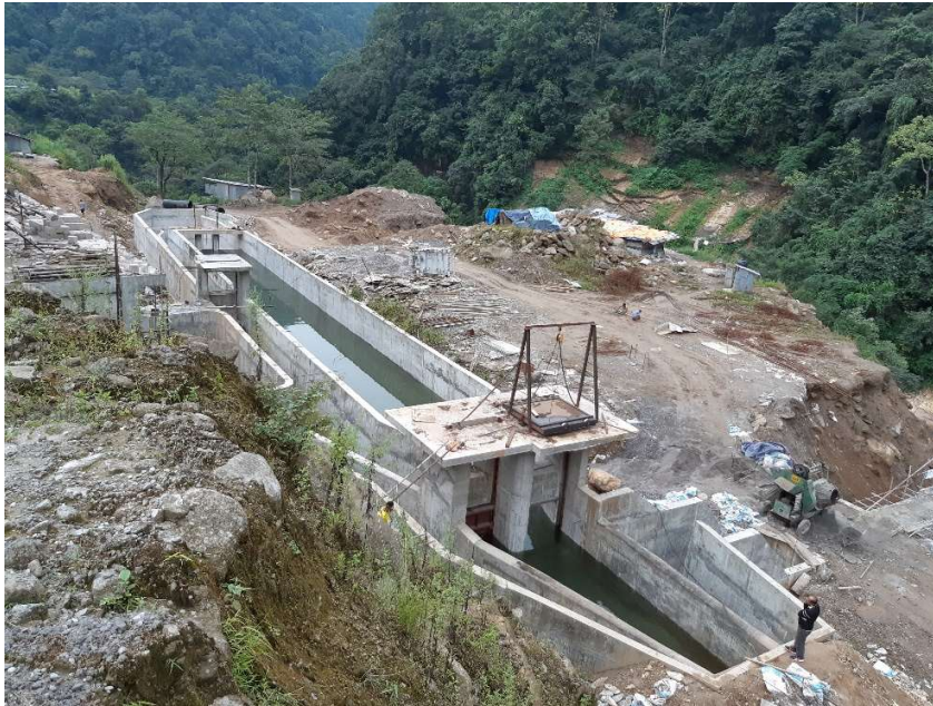
Fig 1: Headpond completed view.
