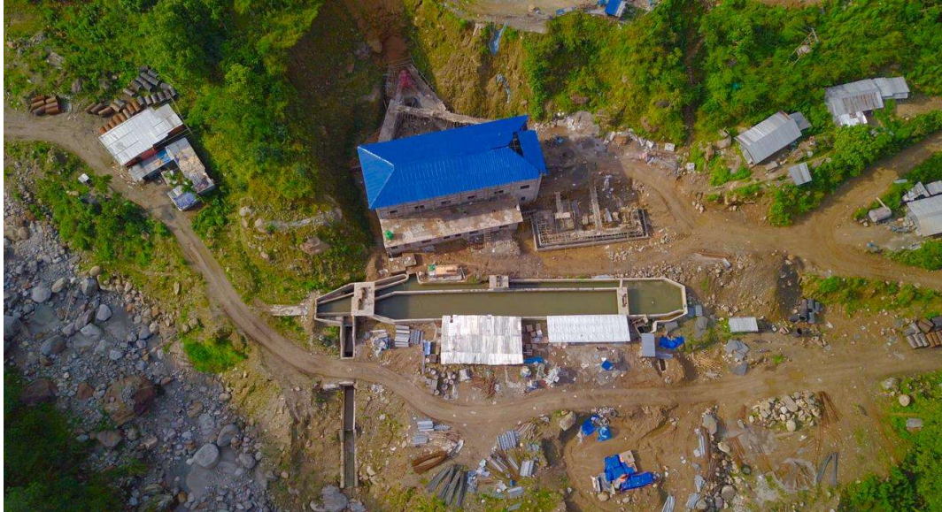
Fig: Headworks area of Rudi A and Rudi B powerhouse.
