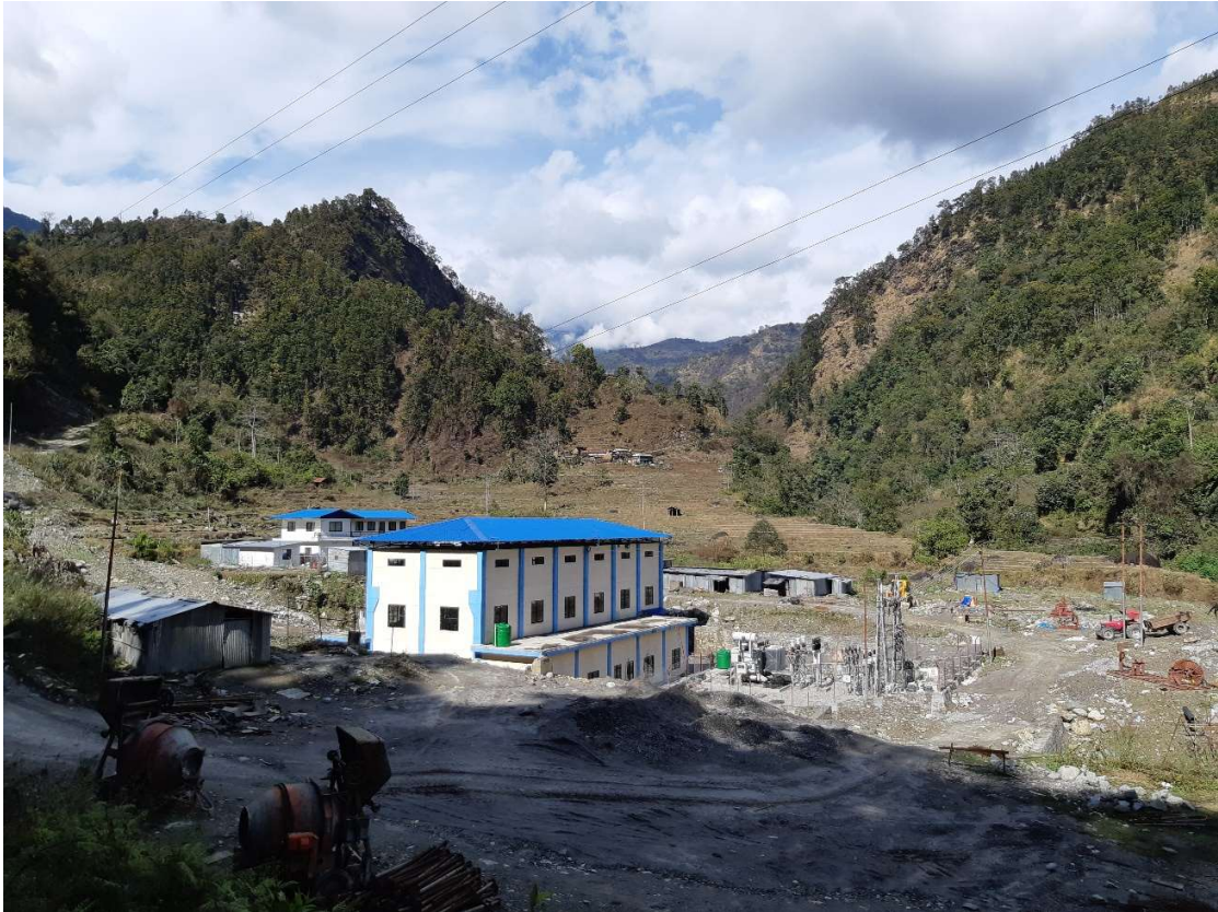
Fig15: Completed view of Rudi A Powerhouse.
