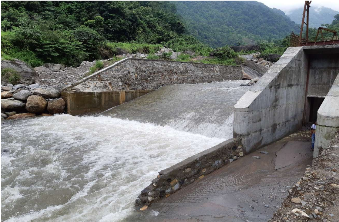
Fig 4: Completed diversion structure with water diverting towards intake.
