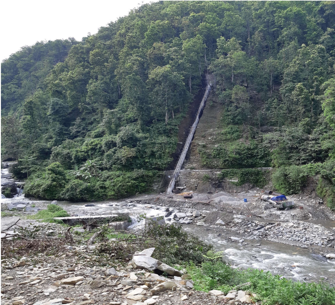
Fig: View of Penstock completed section from patikhola.
